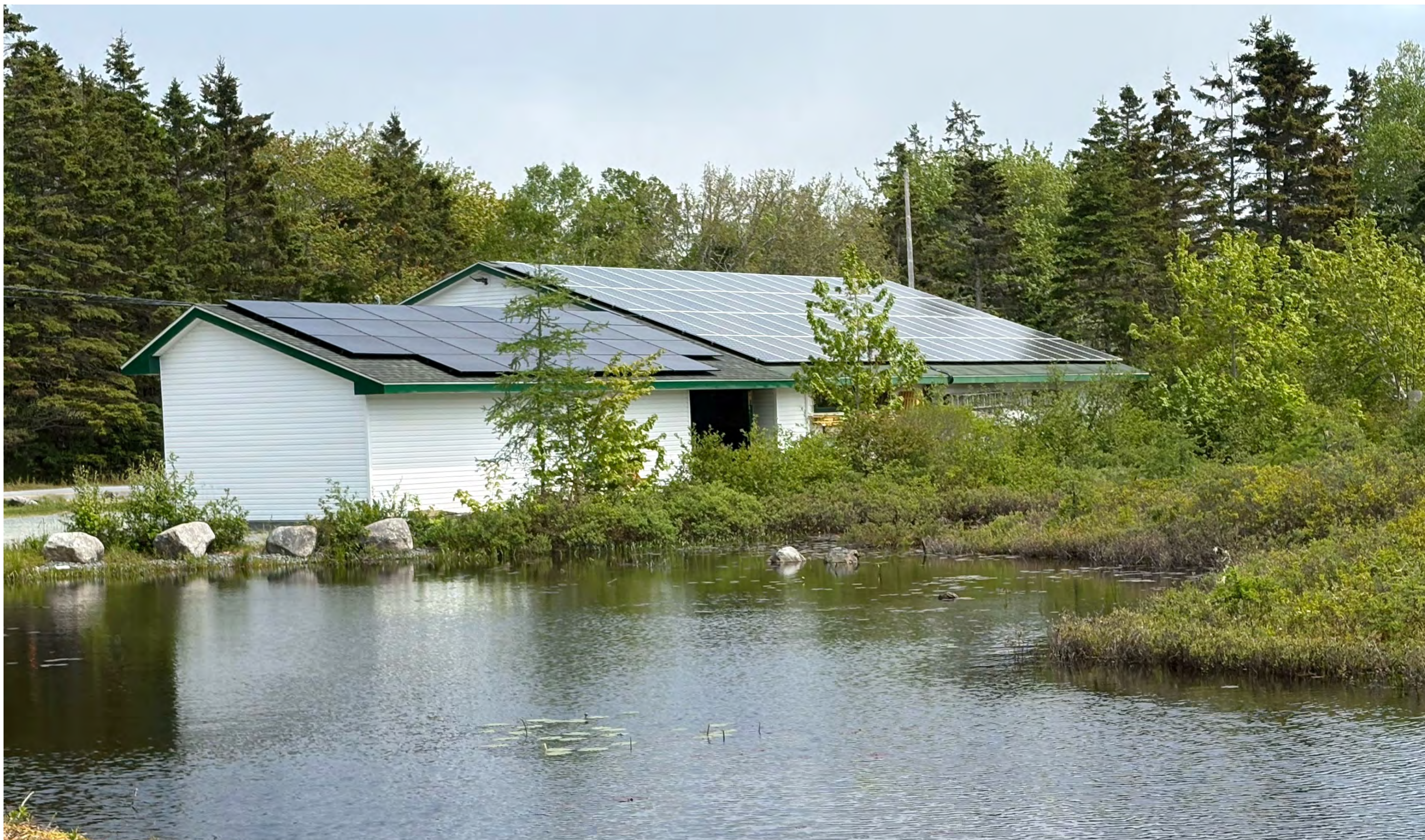
The Memory Lane Heritage Village solar array on the roof of the Artifact Storage Facility/Special Event Equipment Storage Shed (June, 2026)
